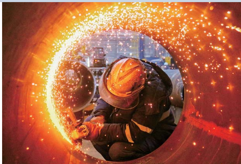
▷ Structural pipe beveling
