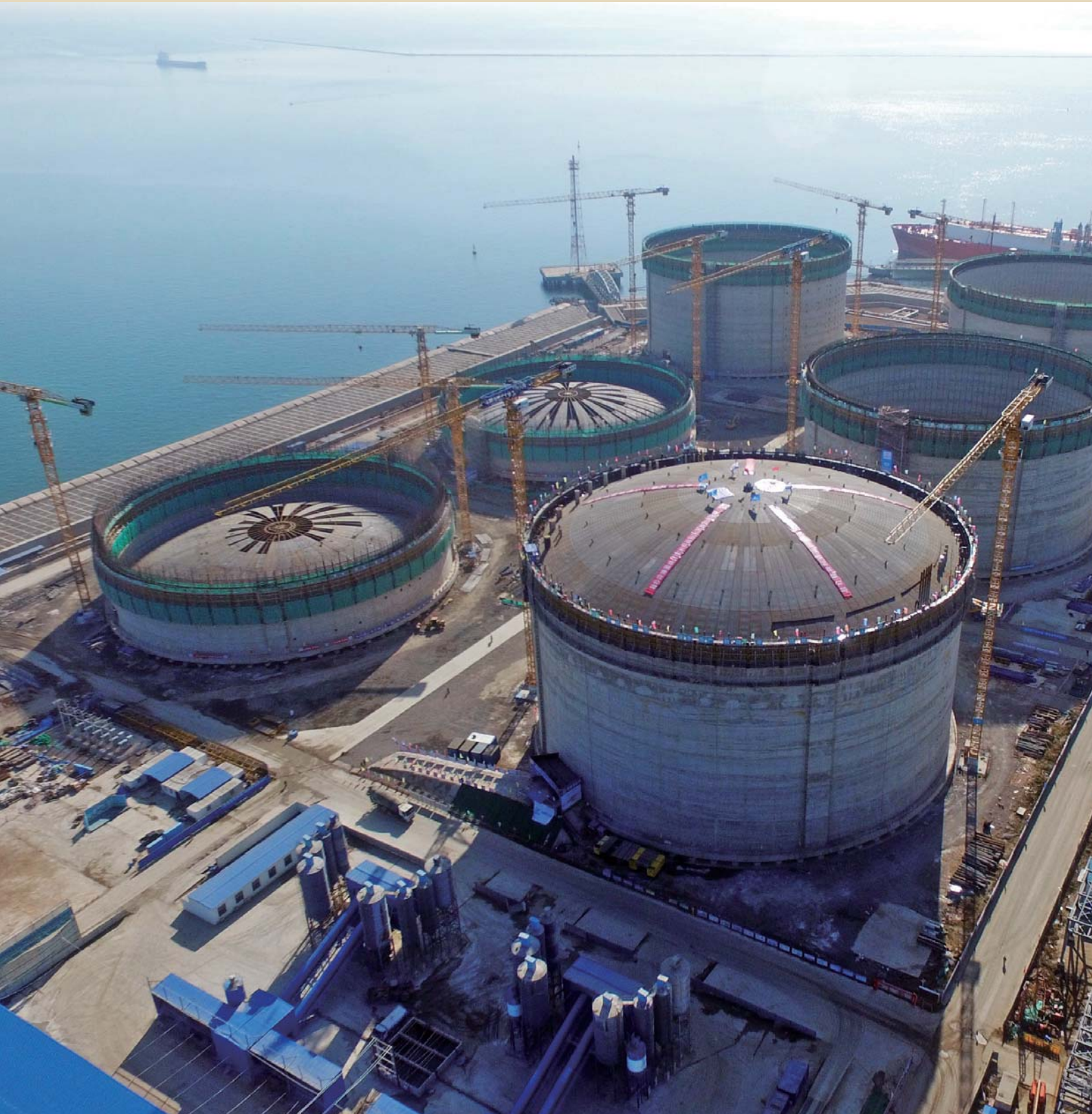
▽ Air raising of the roof of storage tank No. 8, Tianjin LNG Terminal Phase II Project
